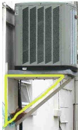
The distinction between professional (safe) and amateur (unsafe) HVAC installations often lies in the quality of these support systems. Designing and fabricating strong shelves, brackets, pipe and duct hangers, suspensions systems, panel supports, guy wire assemblies, conduit systems, raceways, and other underlying components requires a fundamental knowledge of geometry, and almost always involves the Pythagorean Theorem.
